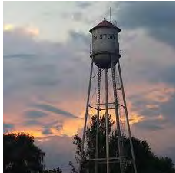
Bristow, Iowa Water Tower
