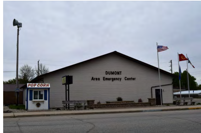
Dumont Area Emergency Center
